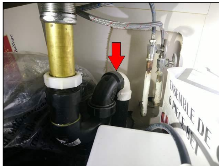
S-trap, venting not visible
