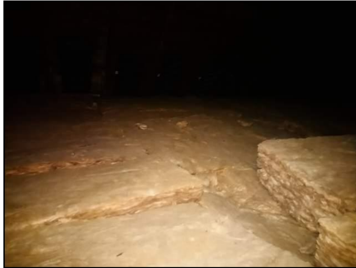
Fiberglass batt attic insulation
