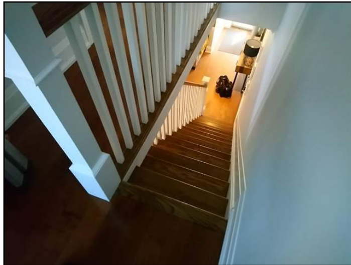
Handrail not continuous to top of stairs
