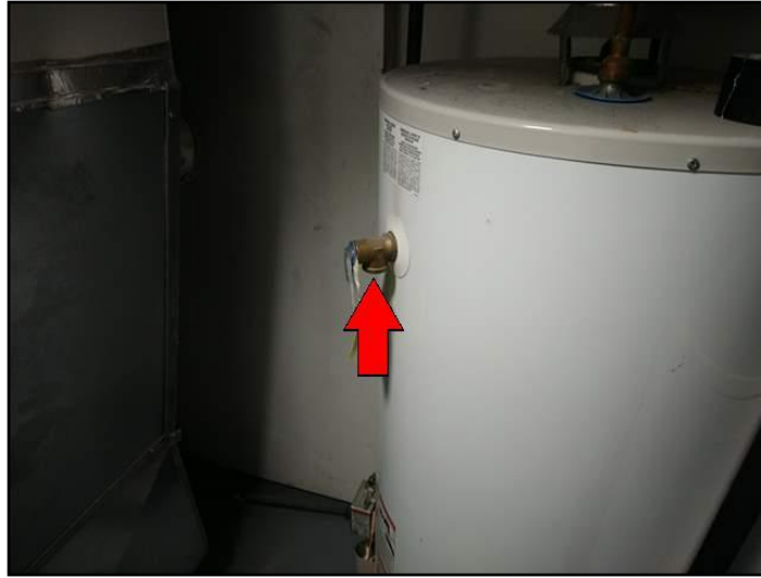
Discharge tube missing
