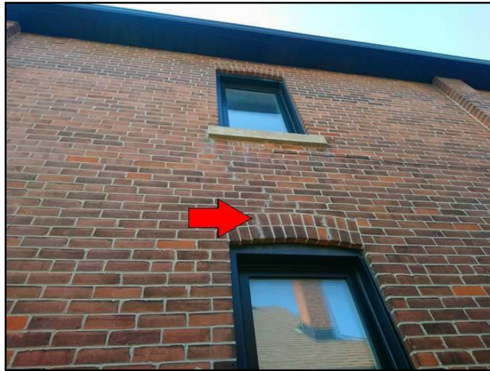
Ex: Minor crack, prior repair noted
