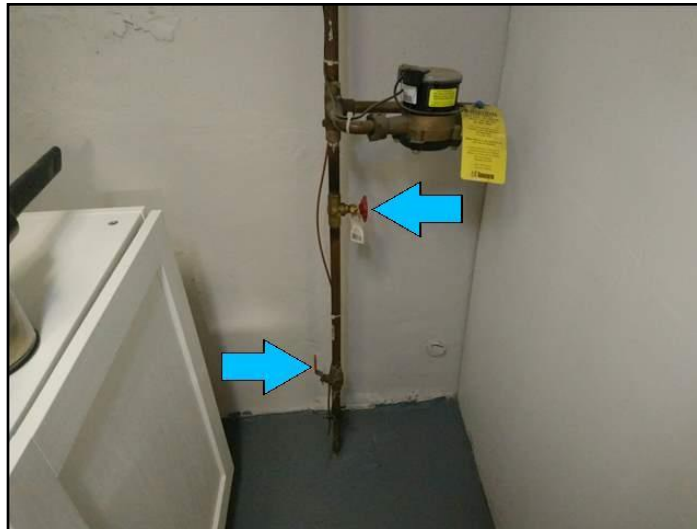
Main water shutoff valve(s)
