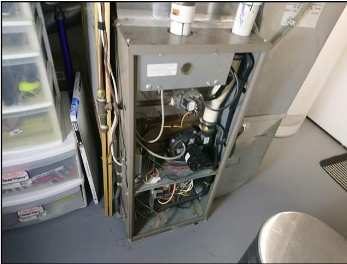
High-efficiency gas furnace
