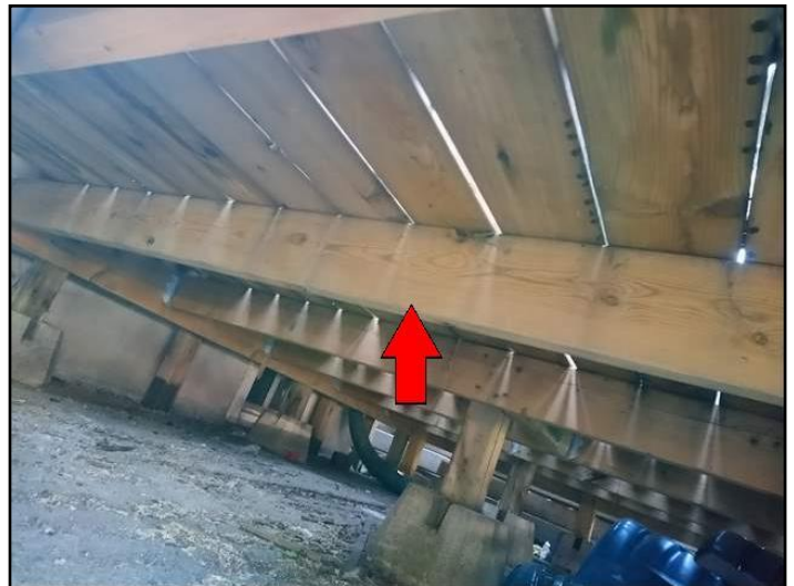
Ex: 2x6 joists noted
