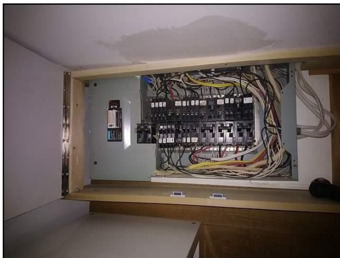
Breaker panel (cover removed for inspection)
