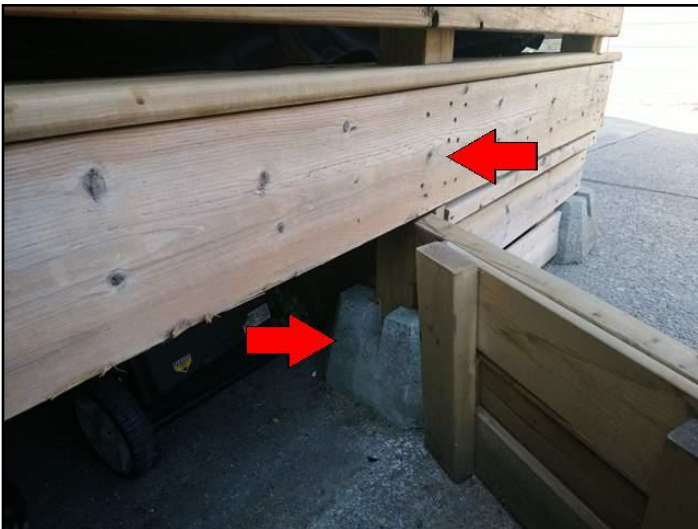
Ex: Missing proper footings; weak connections
