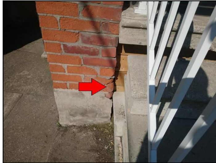
Ex: Spalling
