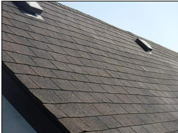
Asphalt shingles (south)
