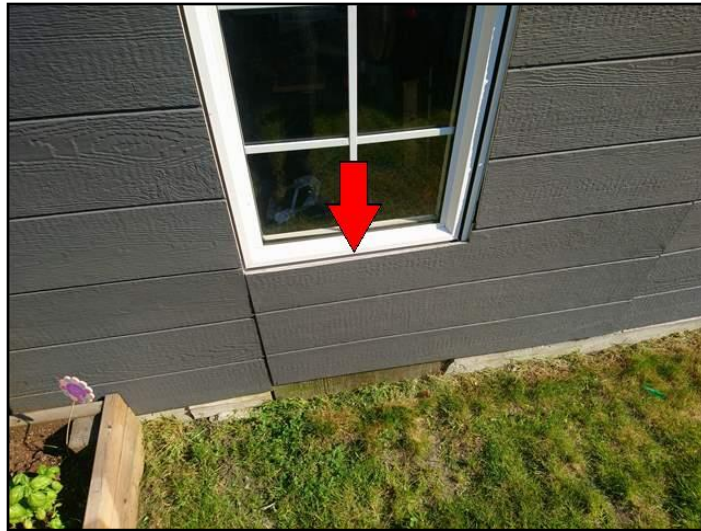
Ex: Not well sealed at window
